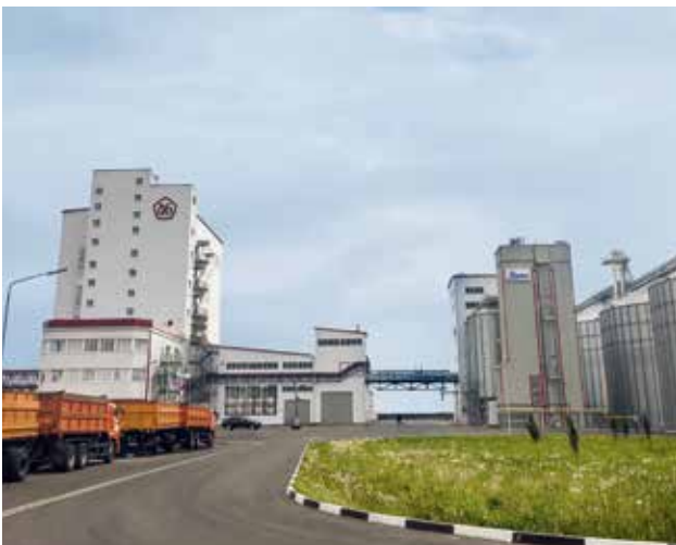
Mischfutterwerk 30 t/h in Belgorod, Russland Compound feed plant 30 t/h in Belgorod area, Russia
