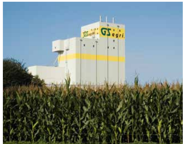
Mischfutterwerk 265.000 t/a in Garrel, Deutschland Compound feed plant 265,000 t/a in Garrel, Germany
