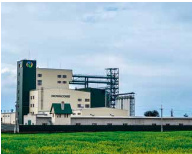
Premix- und Mineralfutterwerk in Dnepropetrovsk, Ukraine Premix and mineral feed plant in Dnepropetrovsk area, Ukraine
