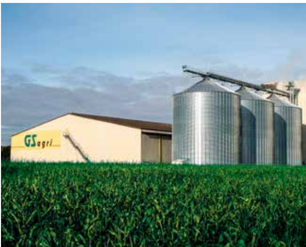
Rundsiloanlage 3 x 4.000 t in Schneiderkrug, Deutschland Storage bin system 3 x 4,000 t in Schneiderkrug, Germany
