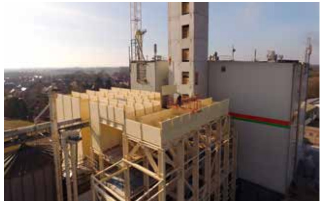
GWS Siloanlagen während Montage | GRP Silo system during assembly
